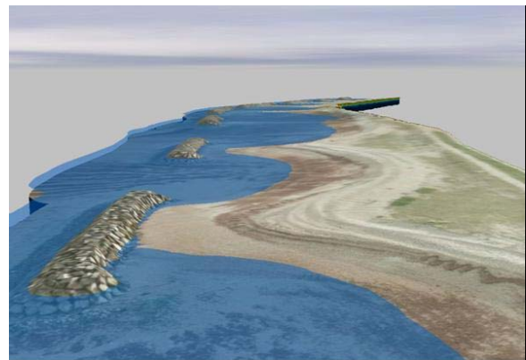
Figure 4 DTM of beach survey at Elmer, overlain with aerial photography
